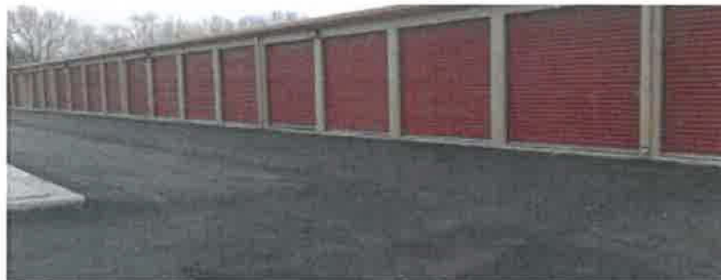
Example of Self-Storage Facilities having numerous garages.
